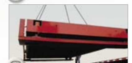
2 Unload and set modules.
