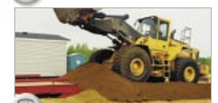
3 Backfill to bulkheads and finish ramps.
